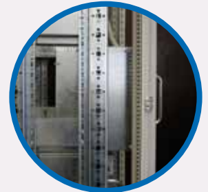
Insertion of the REO-Q modules in the control panel.
